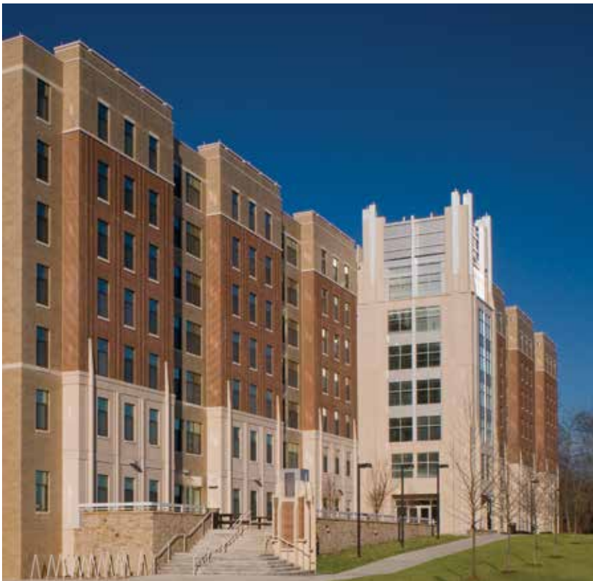
Catholic University's Opus Hall utilized precast concrete sandwich wall panels to create their thermally efficient envelope.
